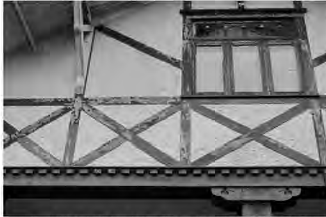
Figure 10 Gable end detailing. Even with severely weathered finishes, the robust detailing of this gable design featuring a stained glass window, a functional soffit bracket, half timbering, a dentiled beam, and a decorative column capital together provide a rich composition.
