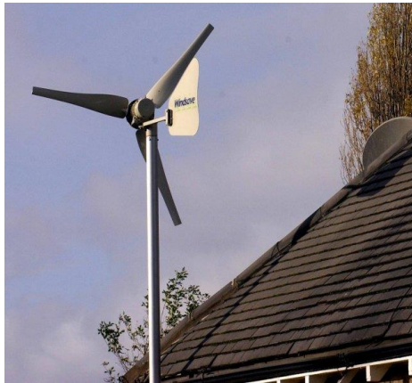
Horizontal-axis wind turbine
