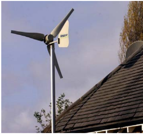
Horizontal-axis wind turbine
