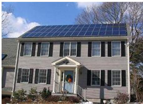
Example of roof-mounted photovoltaic modules.
