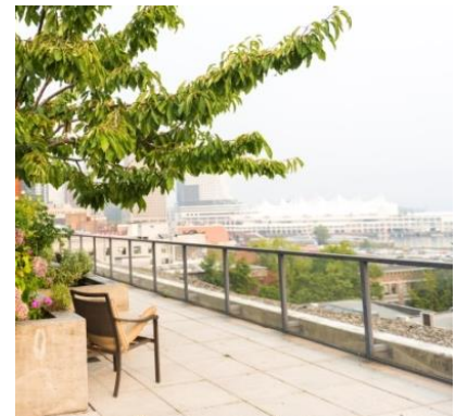
Figure 12. Roof deck guard rails example
