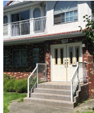
Figure 6. Landing in front yard
