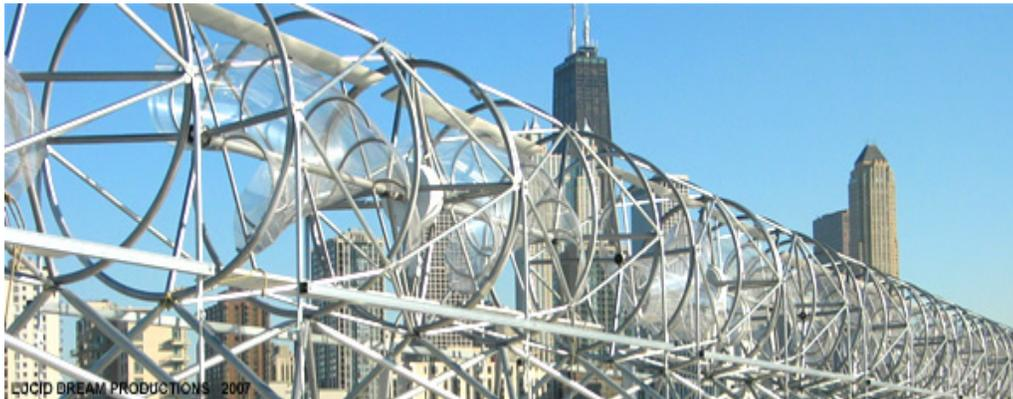
Building-mounted horizontal-axis turbines
