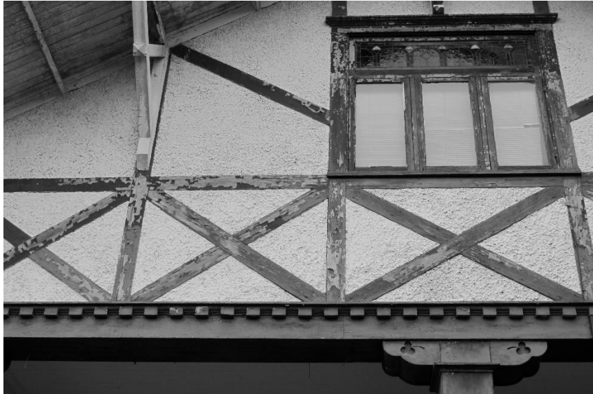
Figure 10 Gable end detailing. Even with severely weathered finishes, the robust detailing of this gable design featuring a stained glass window, a functional soffit bracket, half timbering, a dentiled beam, and a decorative column capital together provide a rich composition.
