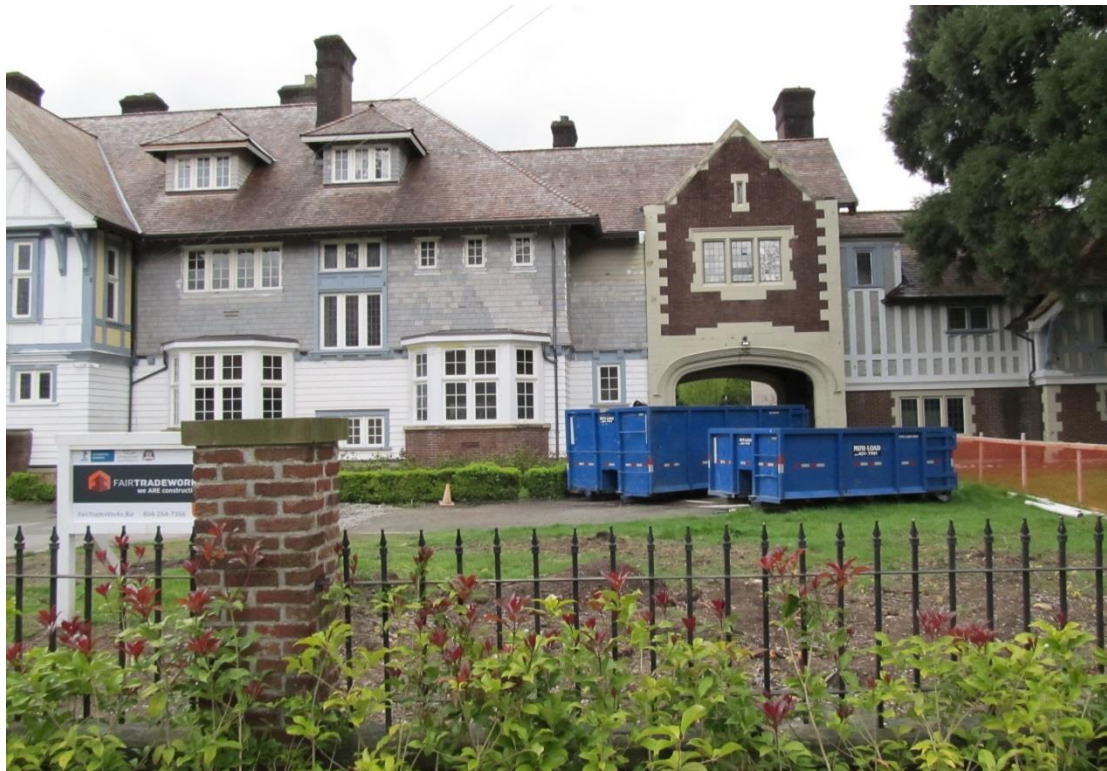
Figure 6 Rosemary, 3689 Selkirk Street, 2015. View from the front yard of the ongoing refurbishment of the exterior cladding.
