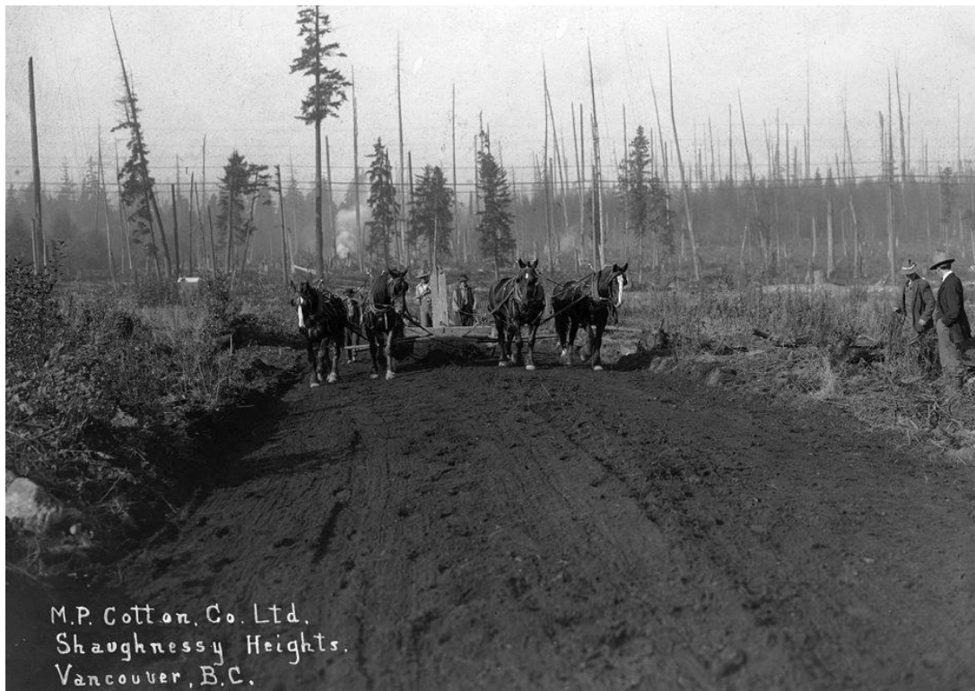
Figure 4 M.P. Cotton Co. Ltd. [engineers and general contractors] road clearing in Shaughnessy Heights, 1911 [City of Vancouver Archives 677-251]
