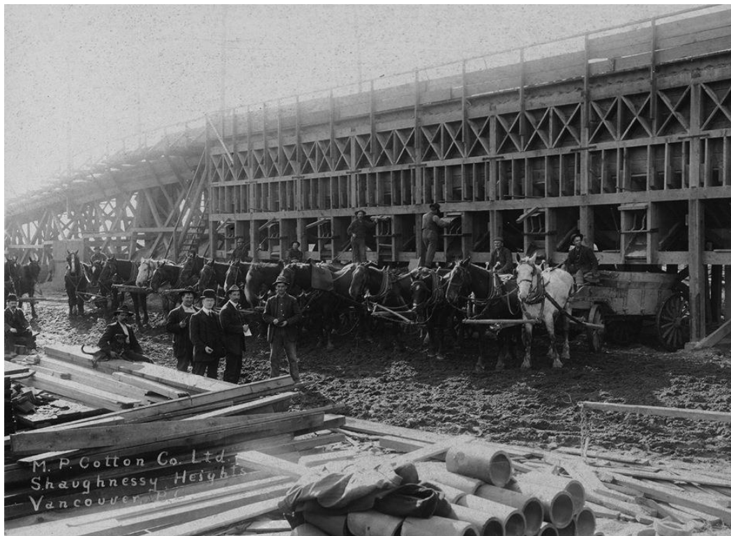
Figure 7 M.P. Cotton Co. Ltd. construction crew and carts in Shaughnessy Heights, 1911 [City of Vancouver Archives Bu P164]
