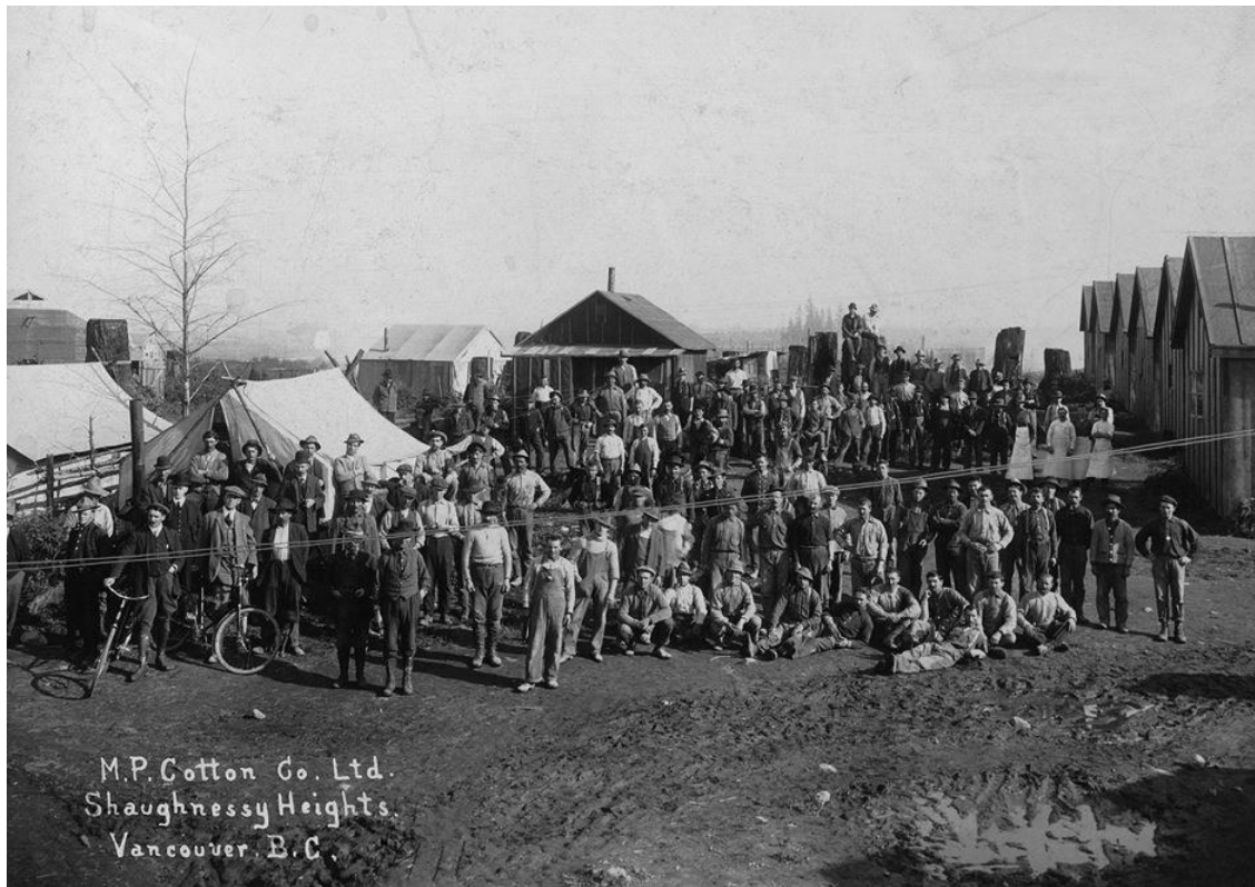
Figure 6 M.P. Cotton Co. Ltd. construction crew and carts in Shaughnessy Heights, 1911 [City of Vancouver Archives 677-249]
